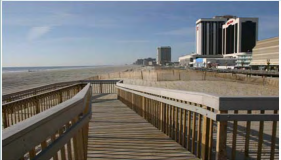
Absecon Island - Completed Handicap Dune Crossing.
