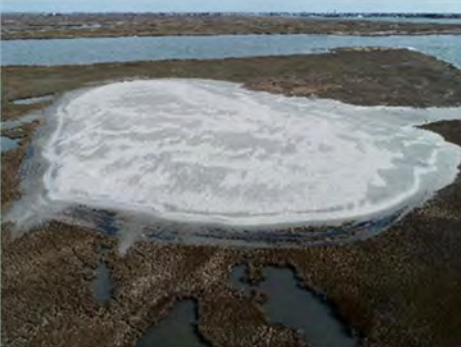
Habitat Creation at Great Flats, near Stone Harbor NJ conducted as part of the NJIWW dredging and beneficial use placement project in December 2018 and again in February 2021. Barnegat Bay Dredging from Harvey Cedars, NJ was contractor for this and several innovative placement projects done through collaboration with the State of NJ.
