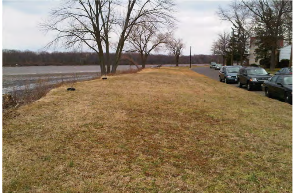
The infrastructure along River Drive in Delran Twp is threatened by erosive forces from Rancocas Creek.
