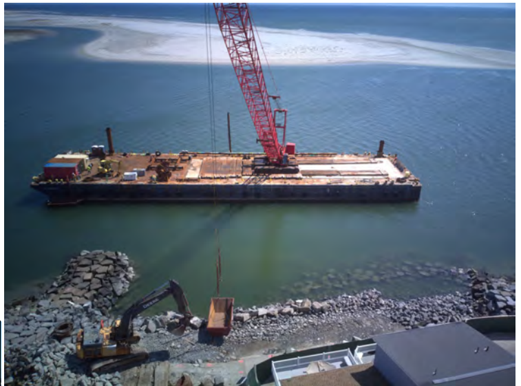
Anglesea Seawall: USACE and its contractor makes repairs to the Hereford Inlet seawall in North Wildwood, NJ in Spring of 2021.
