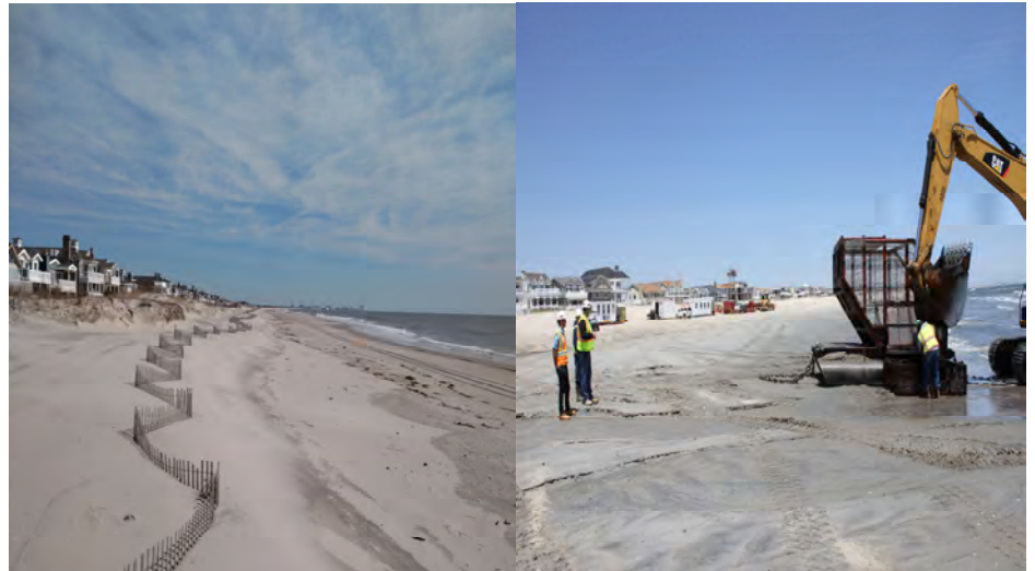
Preconstruction & during construction
