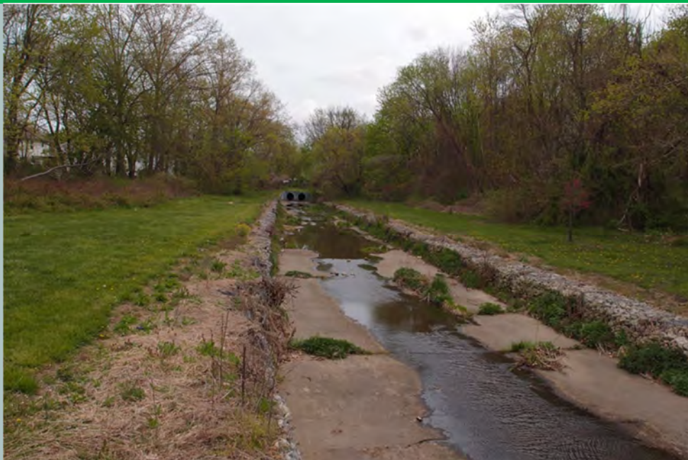
Existing concrete lined channel at Grove Park.
