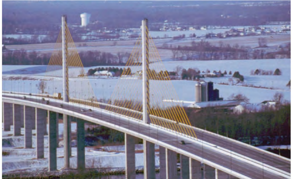
Senator Roth Bridge (SR-1) carrying roughly 34 million vehicles over the C&D Canal per year. Operated and Maintained by USACE Philadelphia District.
