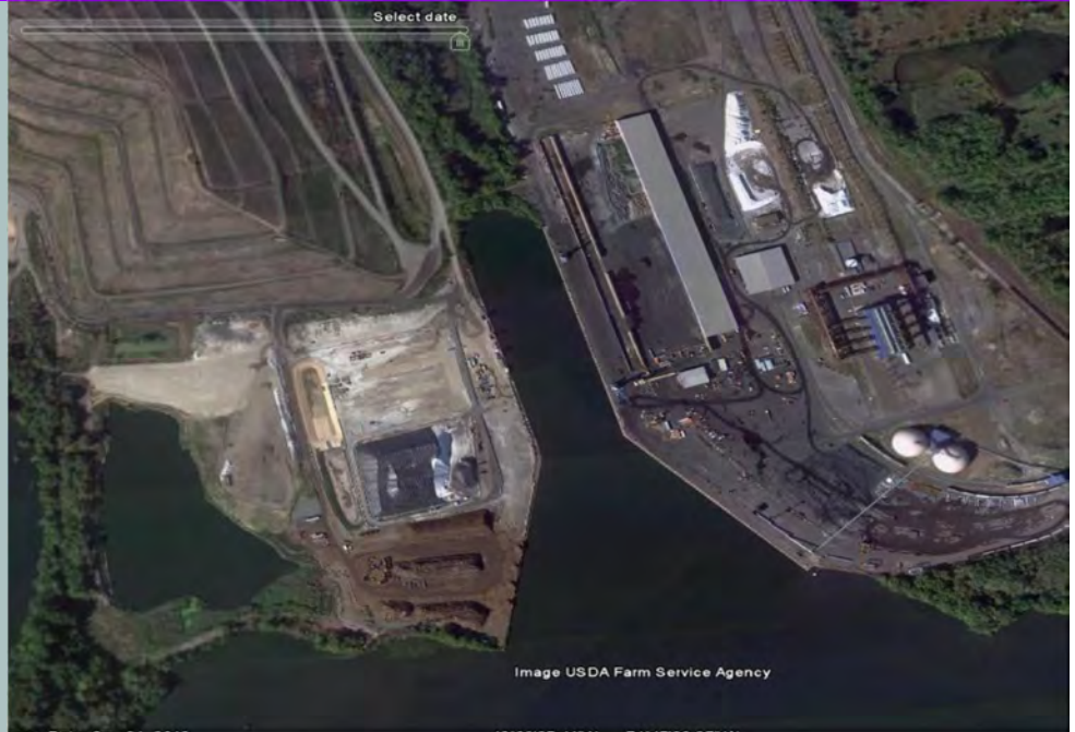
Port of Bucks County—Fairless Turning Basin
