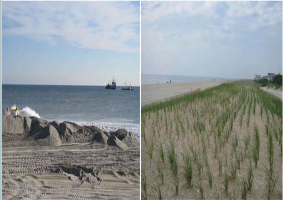
Left: Harvey Cedars Beach fill Initial Construction Right: Harvey Cedars Completed Dune Section
