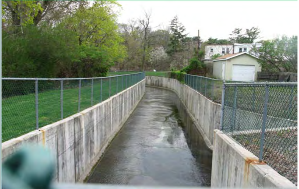
Portions of the creek are channelized in concrete flumes. This might appear to help the problem in one area, but only pushes the flooding problems downstream.
