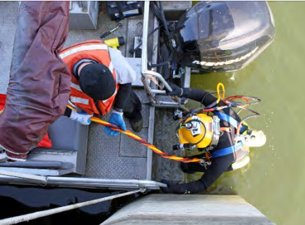
ABOVE: USACE will be making improvements to the upstream embankment of Jadwin Dam in 2022 to reduce risk. LEFT: A member of the District's own Dive Team begins a scheduled underwater safety inspection of the Blue Marsh Dam control tower.
